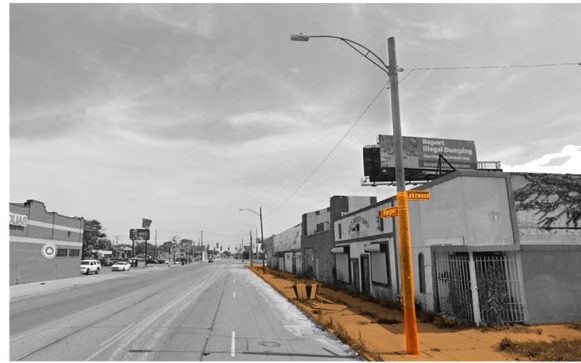
2. Roadside infrastructure such as signboards is poor
