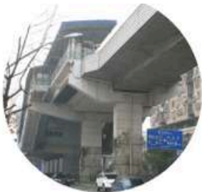
Dazhi Metro Station
